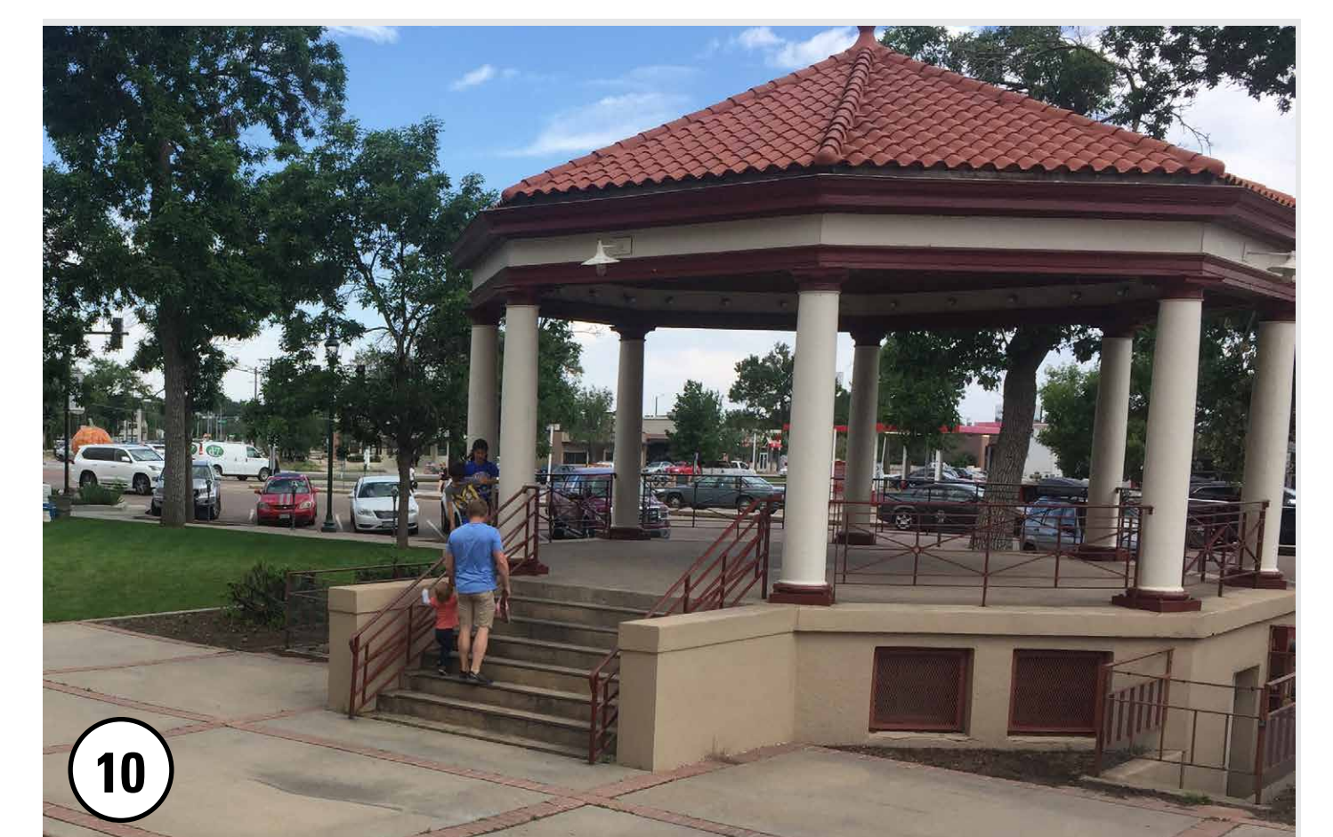
10 Renovations to the historic gazebo will preserve this structure and could include historic interpretive signage.
